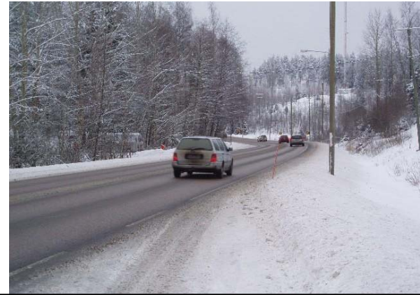
Curve of Koikkala: Road curving on a hill – poor visibility
