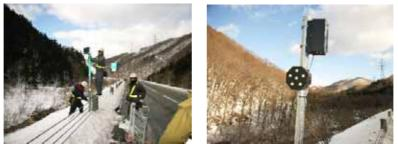
Photo 3. Light emitting delineator equipped with a photovoltaic generator
