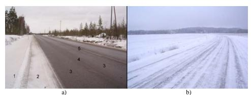
Fig. 4 Friction varies differently across the roads depending on the road type.a) Main road with 1 snow walls, 2 road sides, 3 wheel paths, 4 between wheel paths, 5 between lanes.b) Local road with lower level of service, covered with compacted snow or ice. Friction is generally low all over across the road.
