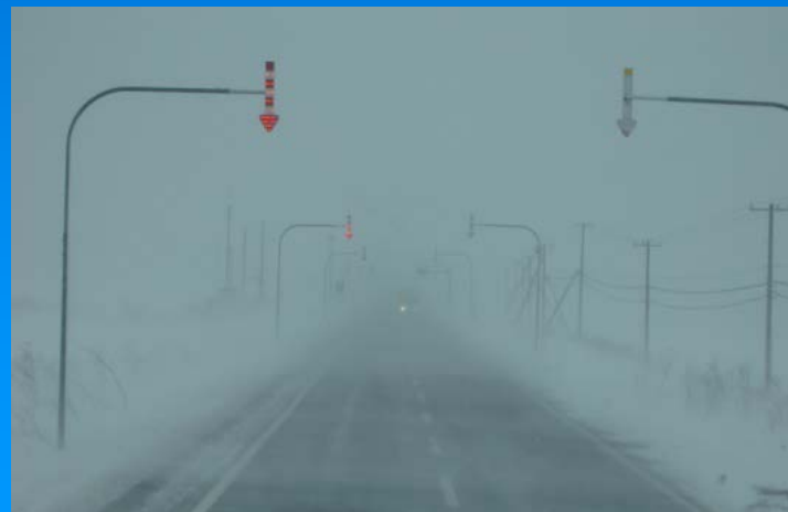
Fixed-post delineators with arrow-shaped pointers
