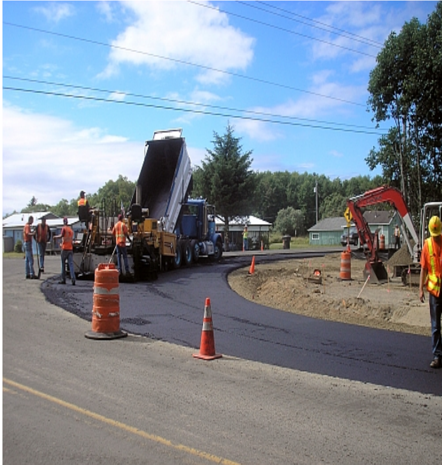
Paving Project, Washington DOT
