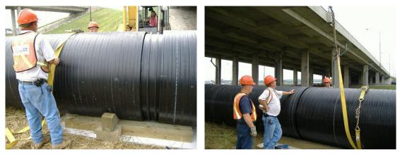
3- Pull in the sections from the first threaded section.
