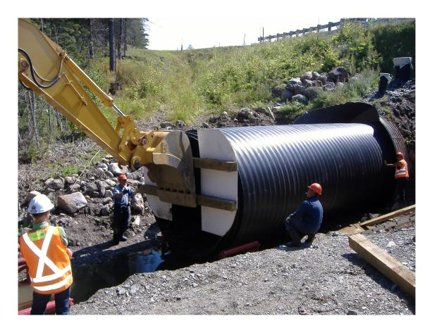
MTQ now have an exhaustive inspection program for their over 62,000 culverts. They have an inspection guide and a method of evaluation. A complete relining specification document that covers all the relining specification including the cement grout mixtures, that is one of the key of the success of this method.
