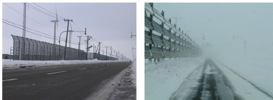
Fig. 2 Snow control facilities (left: collector snow fence, right: blower snow fence)
