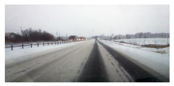
Figure 1. Picture of a road lane section where there are very different road condition in the wheel tracks and inbetween the wheel tracks. There is ice in the wheel tracks and packed snow in-between the wheel tracks.
